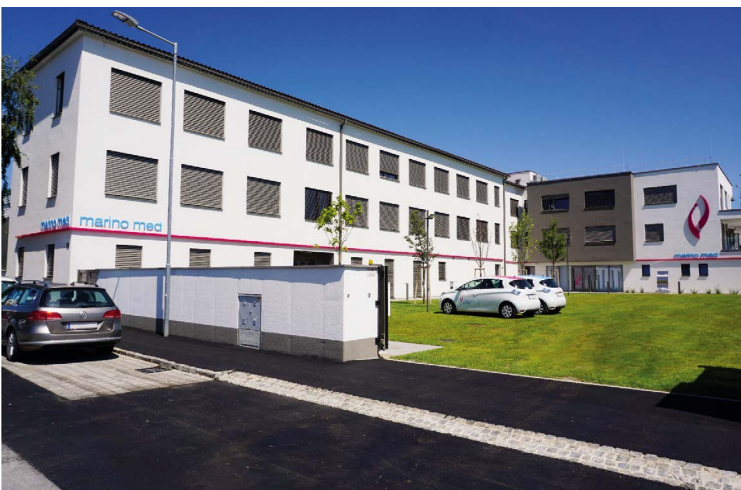
The company premises of Marinomed Biotech AG before the acquisition and conversion of the property in July 2019 (above) and after the conversion work was finished in July 2021 (below). A large part of the existing buildings were removed and the area was unsealed. The existing office building (left part of building) was thermally renovated and an environmentally friendly new building was built at the back of the property. The car park was laid out as a drainage-capable gravel lawn and has charging stations for electric vehicles.
